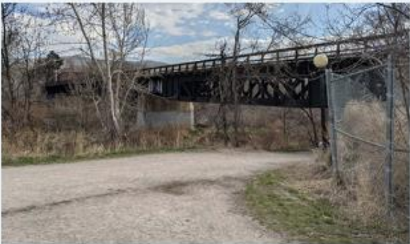
Existing Montana Rail Link Trestle
